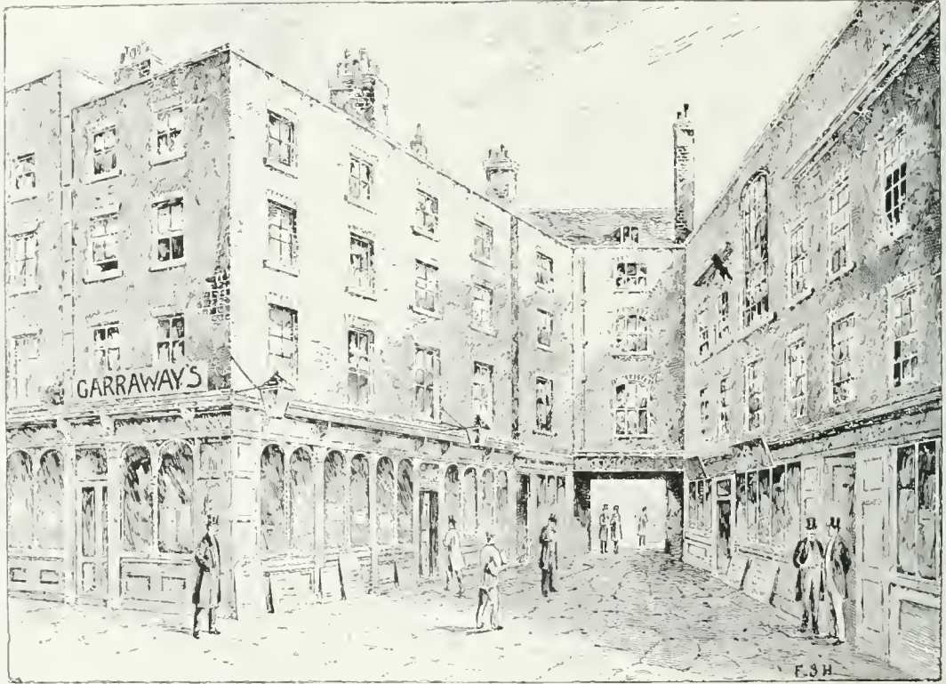
"GARRAWAY'S" SHORTLY BEFORE DEMOLITION ( p. 199).
